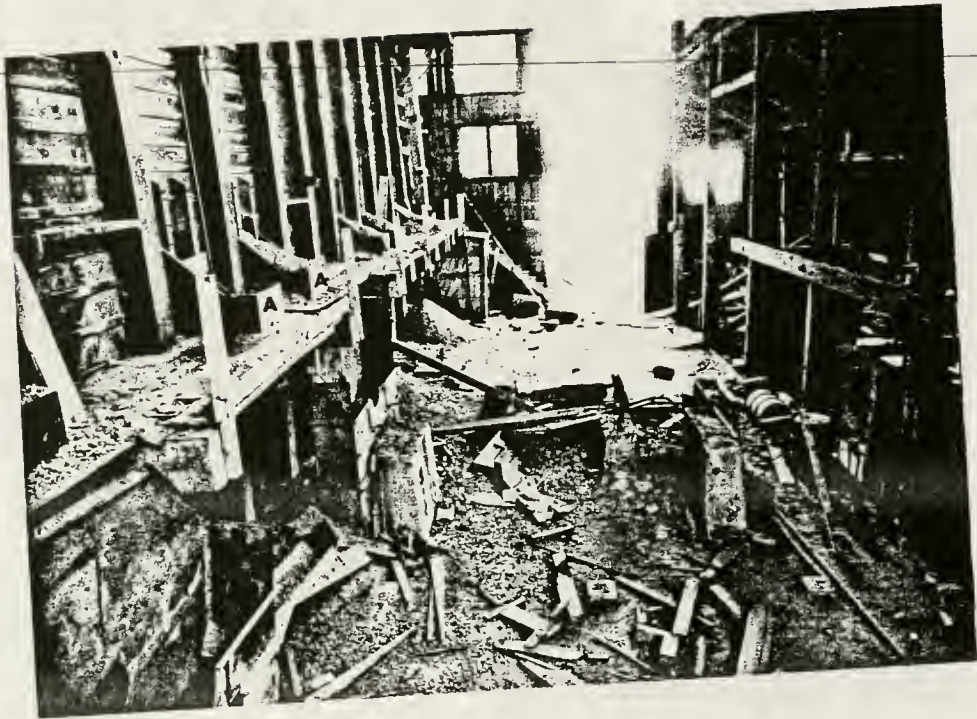
Figure 94. Revenue Mill (structure #34) interior view looking south that shows shoots (A) that fed into ball mills (B).
